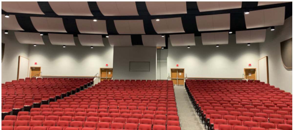
New acoustical ceiling featuring curved reflectors
